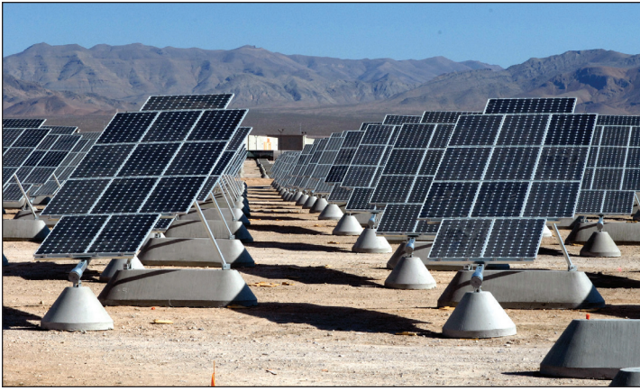
The Nellis Solar Power Plant is located within Nellis Air Force Base in Clark County, Nevada, northeast of Las Vegas. the Nellis solar energy system will generate in excess of 25 gigawatt-hours (90TJ) of electricity annually and supply more than 25% if needed power used at the base.
