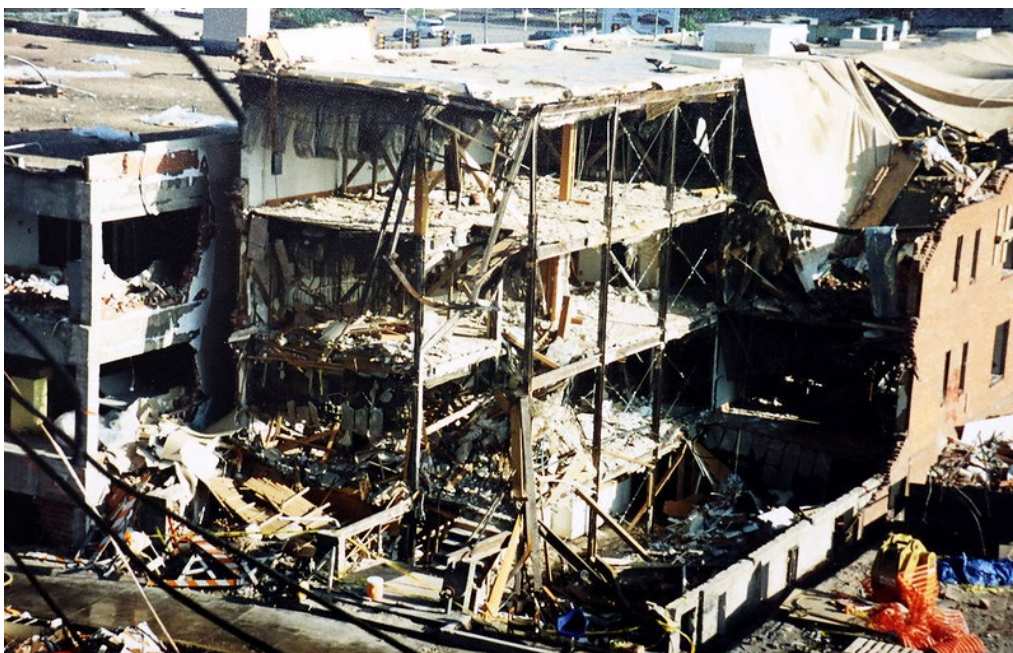
The Alfred P. Murrah Federal Building in Oklahoma City, April 19, 1995, bombed using HME. By usacetulsa (CC BY 2.0).
